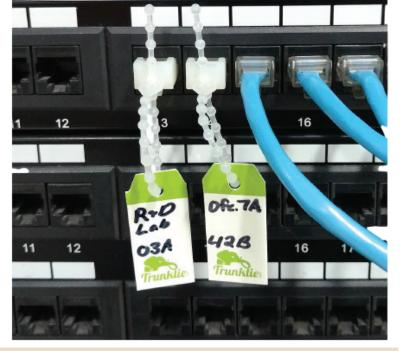
Trunkties plug into an unused RJ45 port, with a flexible and adjustable wrap that secures a Trunktie label tag.
